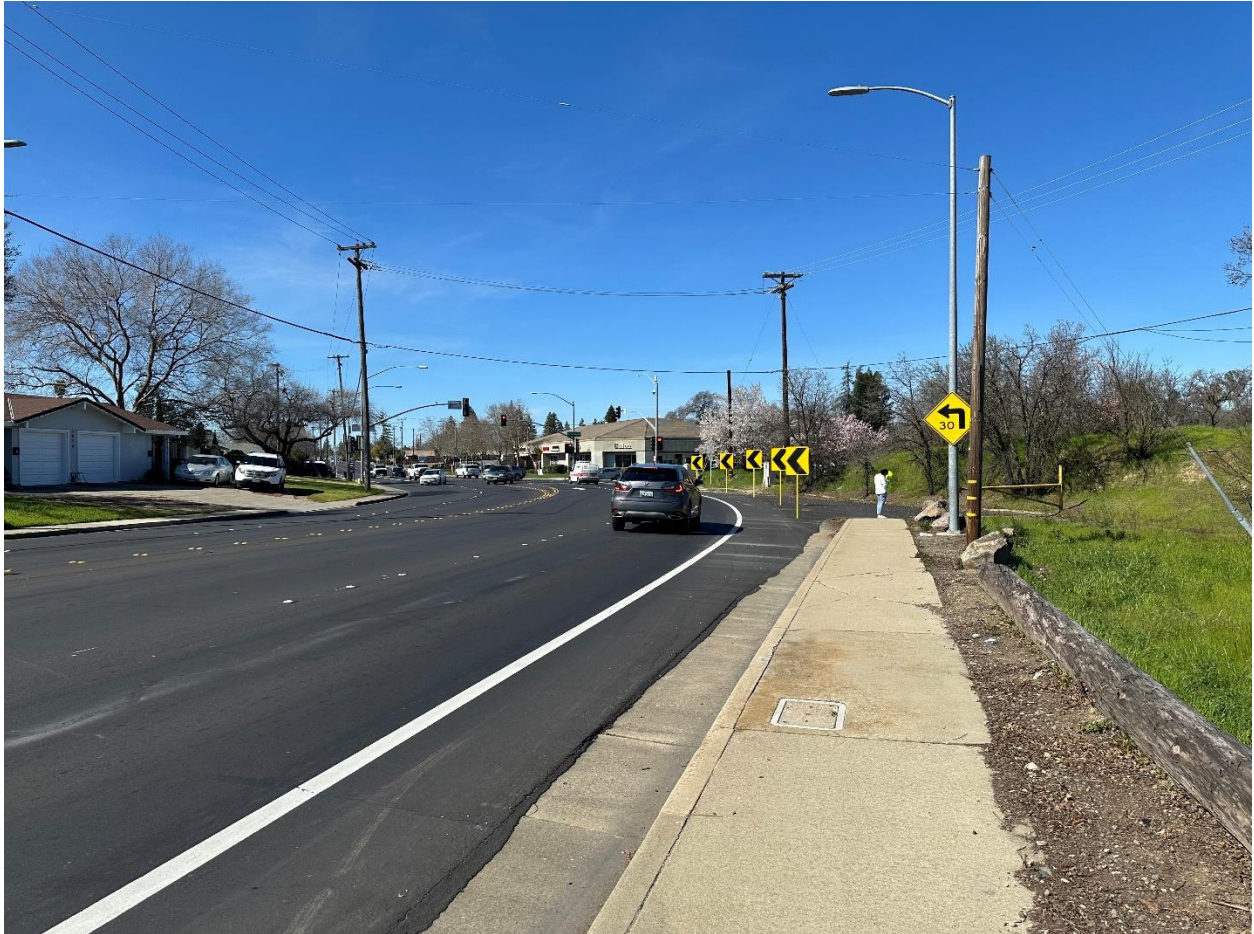
Image 1: Sidewalk gap and advisory chevron alignment signs on Cirby Way.
