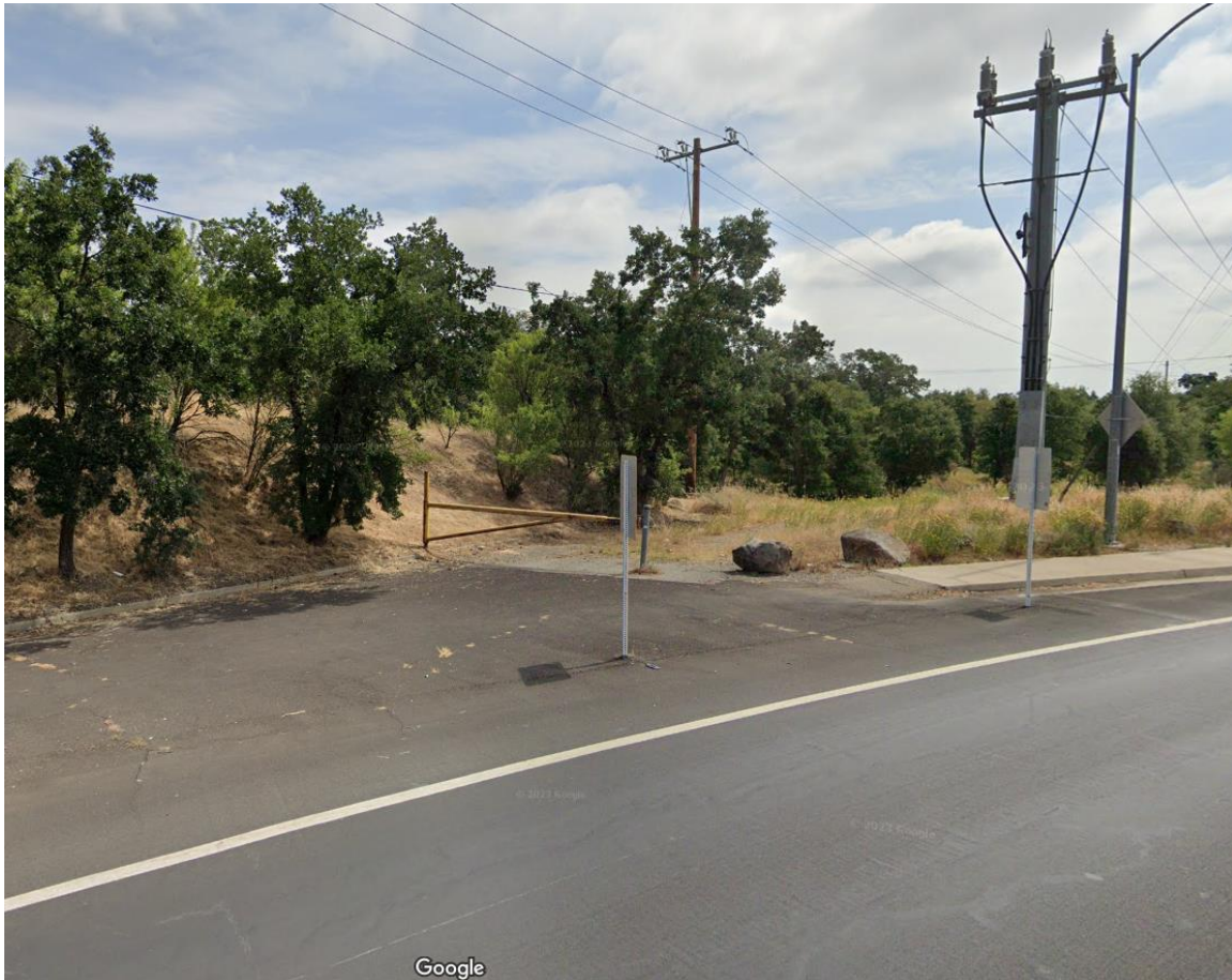
Image 5: Existing gate on Cirby Way at the proposed location of Driveway 2.
